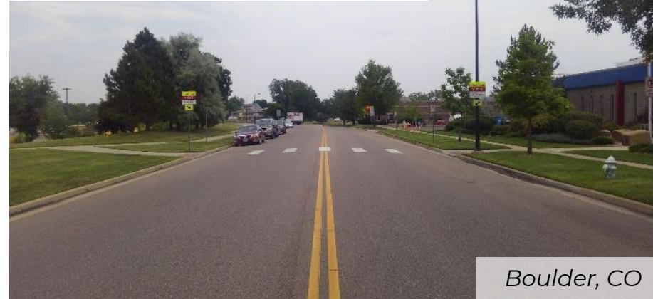
Before Quick Build
