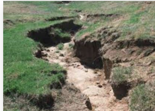
Erosion and Siltation Control
