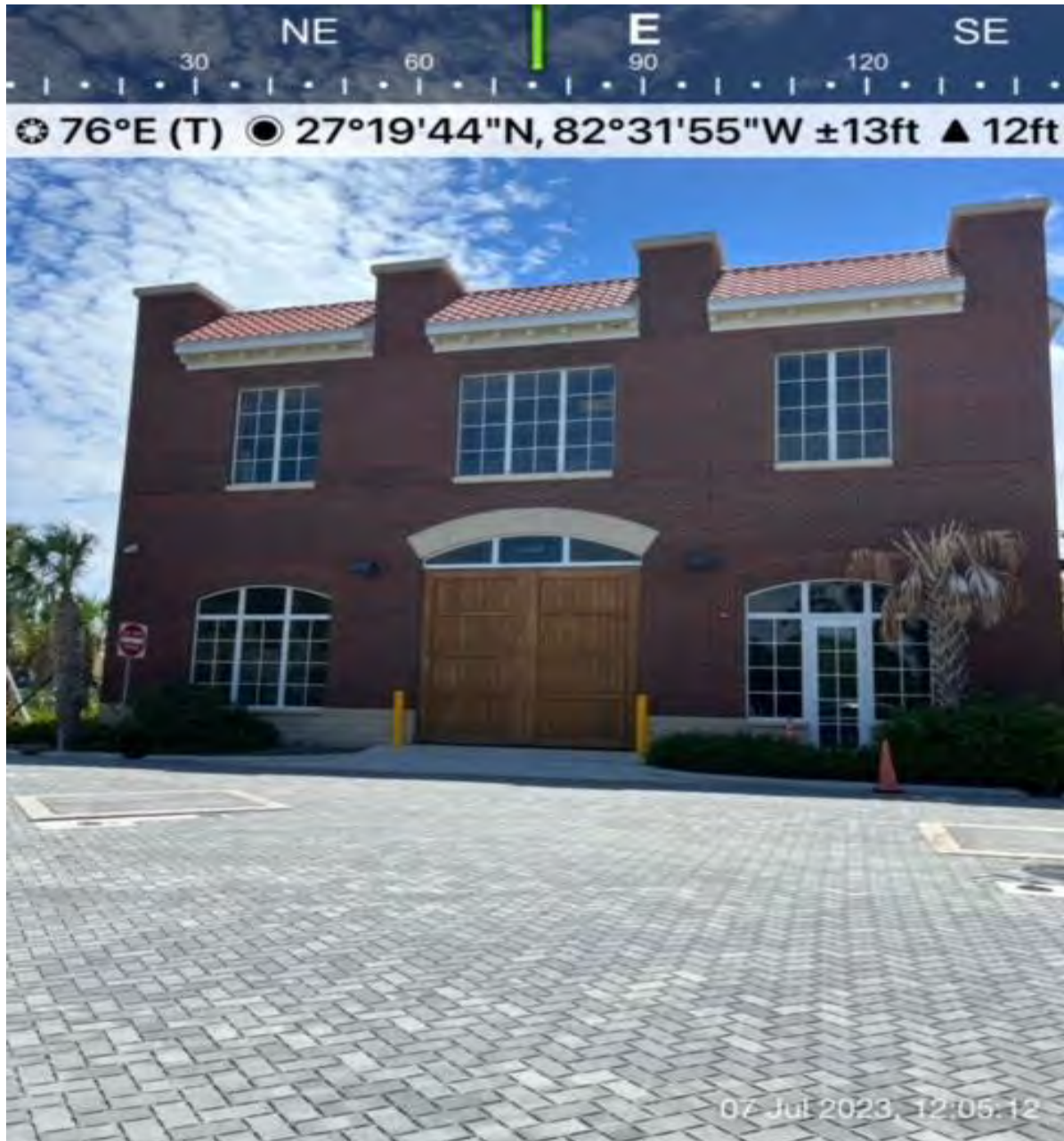
Site #3: City of Sarasota Lift Station (LS) #87 1900 Mound Street, Sarasota, Florida Date of Field Review: July 7, 2023 Front driveway of Lift Station, facing east
