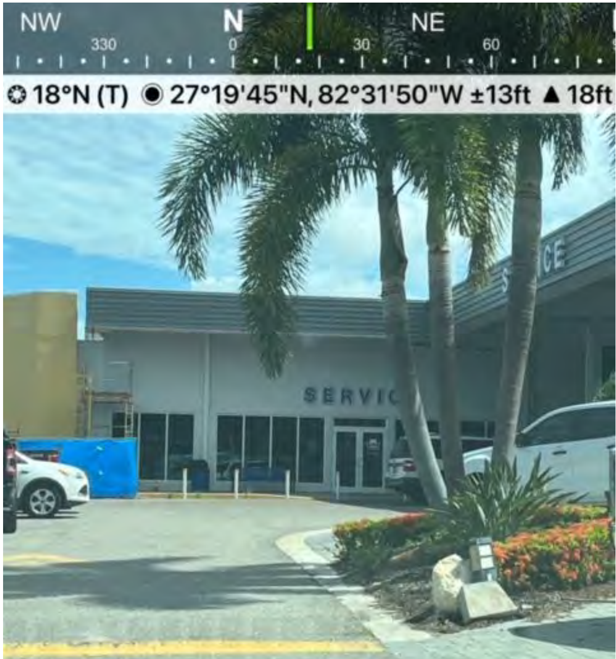
Site #2: Sarasota Ford 500, Inc. 707 S. Washington Blvd., Sarasota, Florida Date of Field Review: July 7, 2023 Service Department, facing north-northeast
