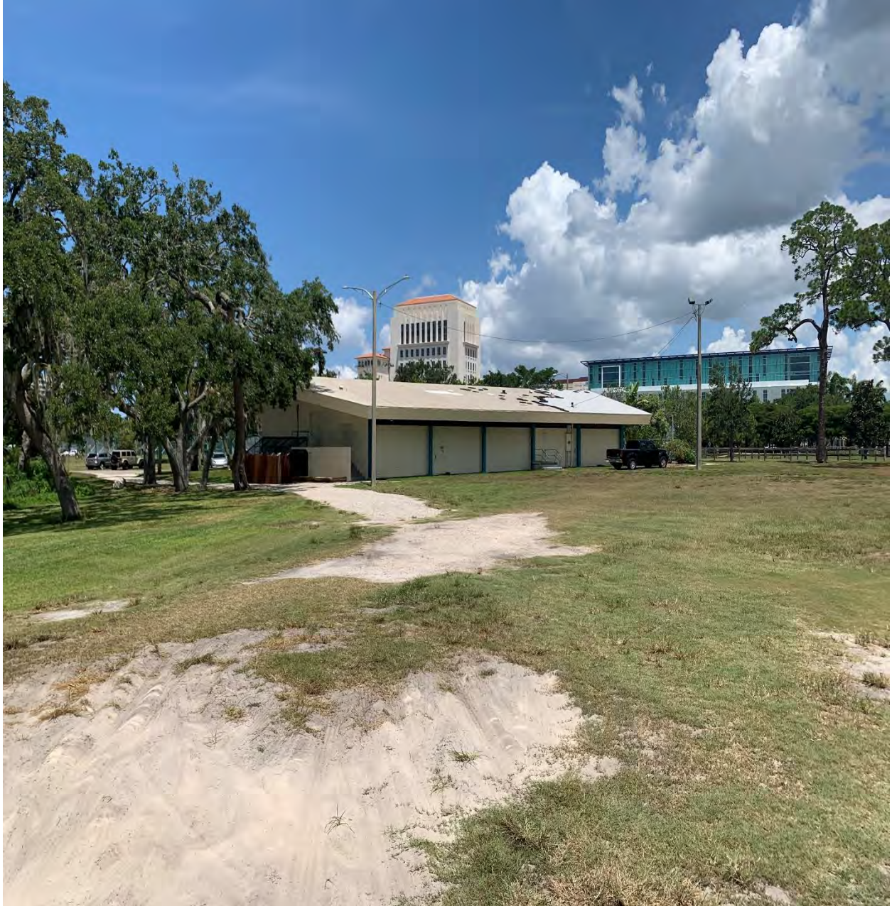
Site #5: Sarasota Mobile Home Park 2100 Laurel Avenue East, Sarasota, Florida Date of Field Review: August 4, 2023 East side of Auditorium in Payne Park, site of former UST/ASTs, formerly part of Sarasota Mobile Home Park, facing northwest
