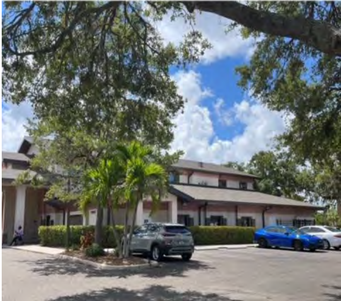
Site #1: Senior Friendship Centers 1820/1900 Brother Geenen Way, Sarasota, Florida Date of Field Review: July 7, 2023 Building onsite, facing northeast
