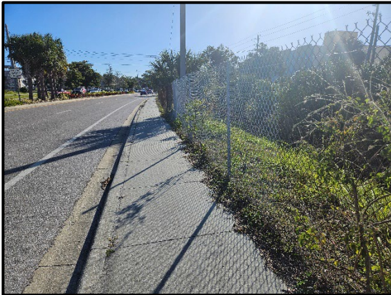
Photo 2.11. Chain link fence adjacent sidewalk along south side between Lemon and Orange Avenues, facing east.
