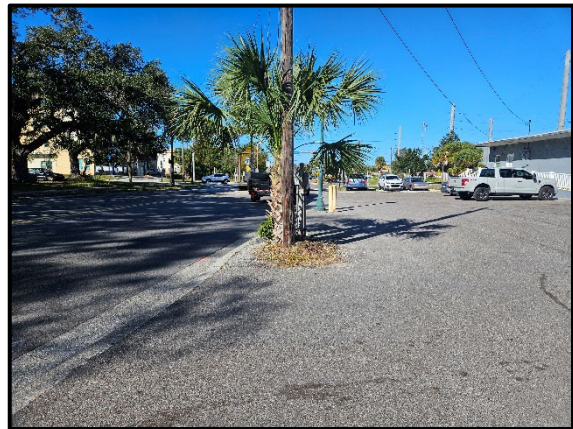
Photo 2.14. Conditions of north side of 10 th Street east of Orange Avenue intersection in east project terminus, facing west.
