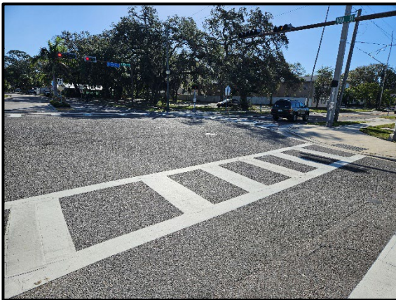
Photo 2.13. South side of Orange Avenue/10 th Street intersection, facing southeast.
