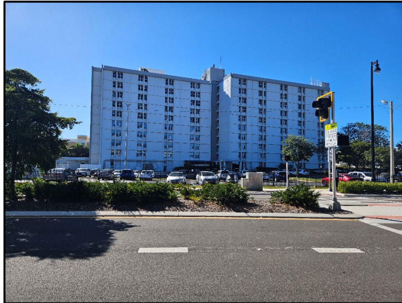
View of northern portion of 8SO00041 (destroyed) within the project limits, now the location of the Jefferson Center retirement facility adjacent to the south side of 10 th Street, facing south.
