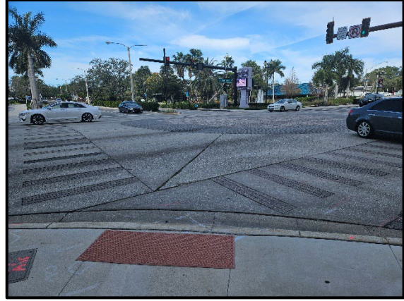
Photo 2.4. View of US 41/Blvd of the Arts intersection from southeast corner, facing northwest. Note utility markings.
