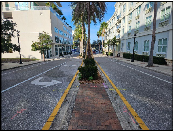
Photo 2.5. Conditions of Blvd of the Arts toward US 41 from west of Coconut Avenue, facing west.
