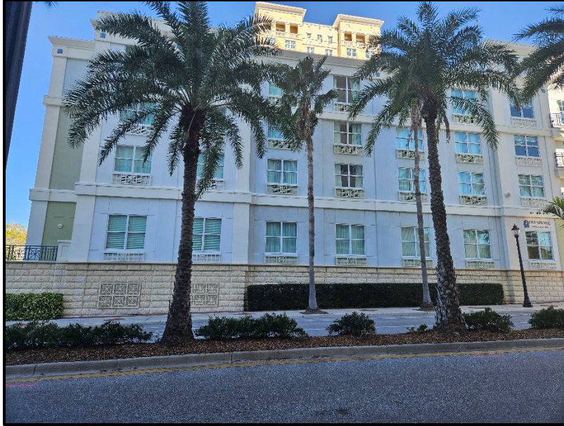
Photo 5.3. View of southern portion of 8SO00041 (destroyed) within the project limits, now the location of Voco Sarasota Hotel adjacent to the north side of Boulevard of the Arts, facing north.
