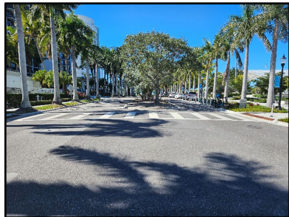
Photo 2.2. Conditions of west project terminus towards Sarasota Bay at Van Wezel Way, facing west.
