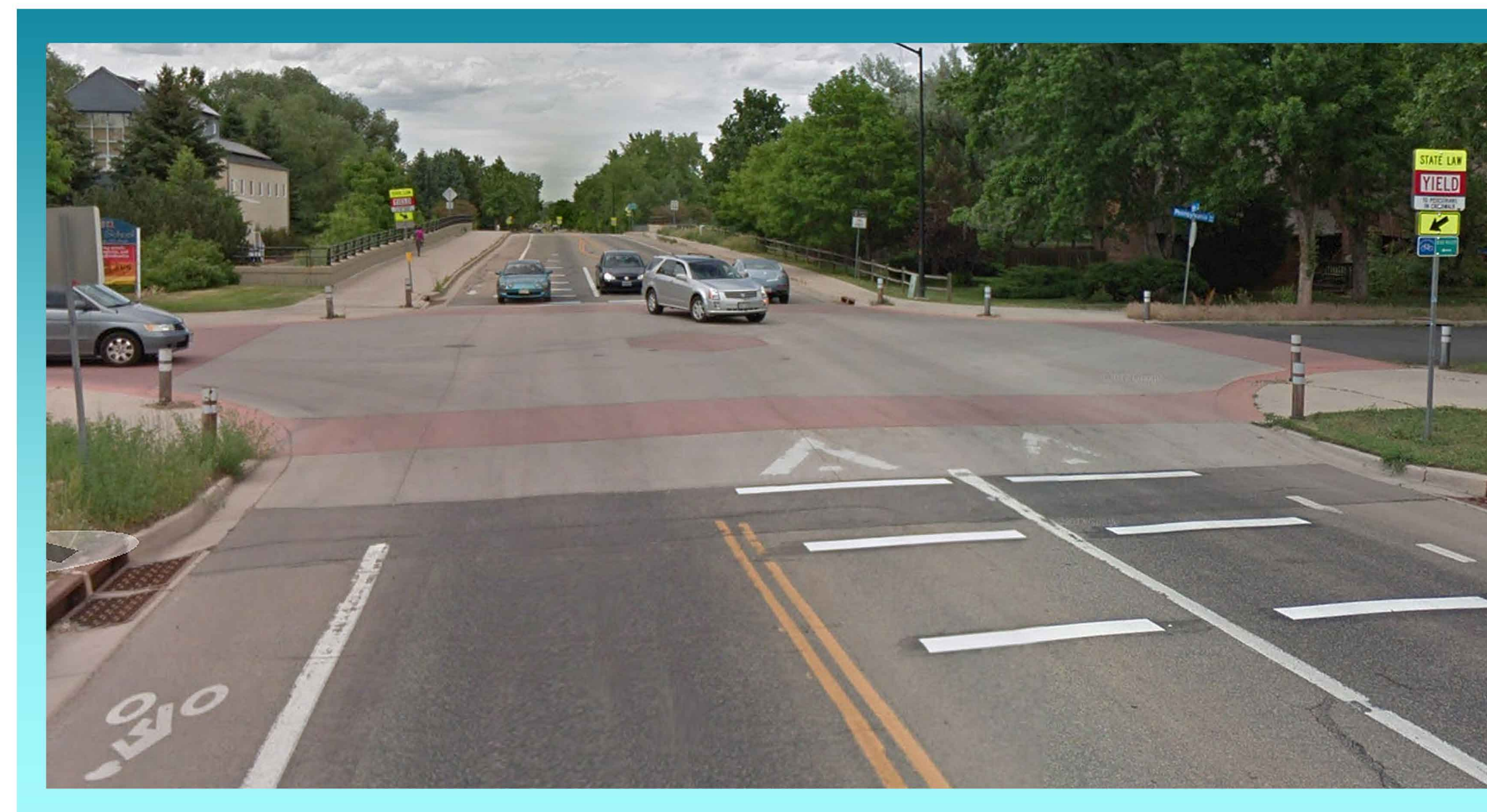
Raised intersection safety treatment from Boulder, Colorado
