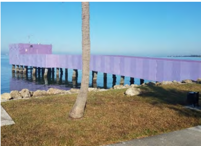
(Bottom): City of Sarasota Wastewater Treatment Plant
