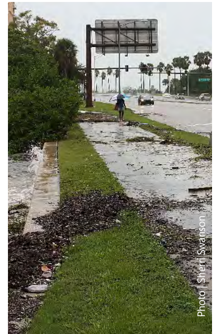
Gulfstream Drive (SR789) Storm Surge Debris following Hurricane Hermine
