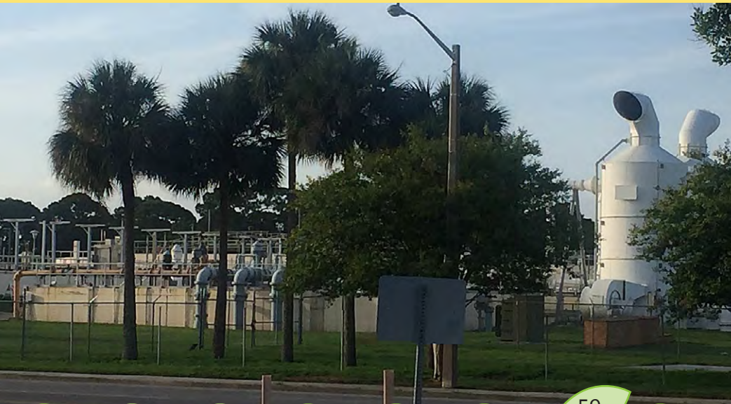
(Top): Sanitary Sewer Overflow August 27, 2017 Extreme Precipitation Event
