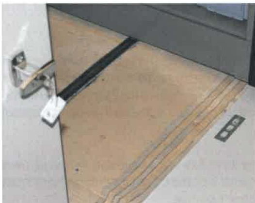
Property and Evidence shelving locks
